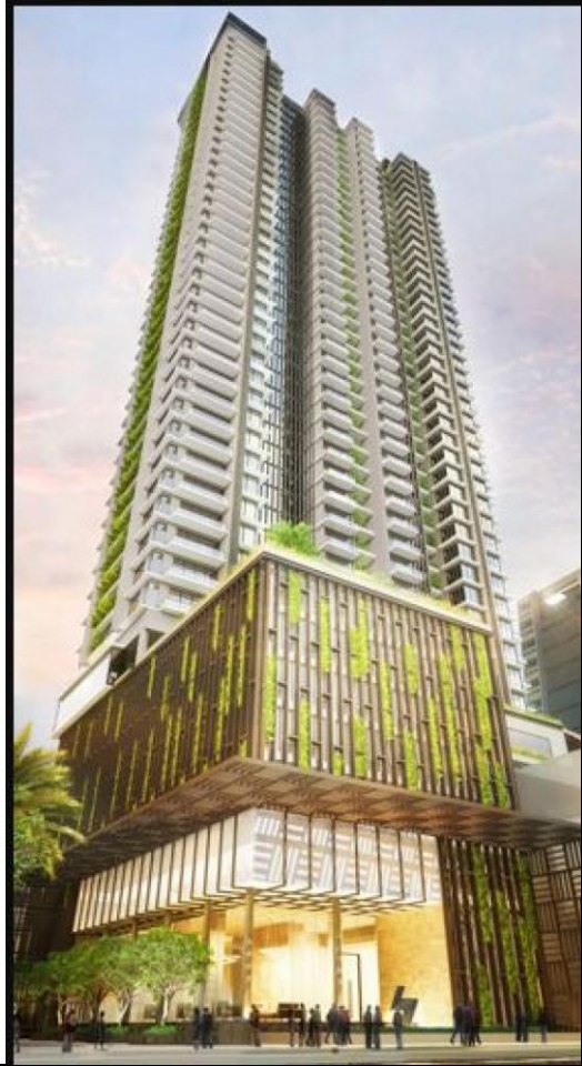
Union Apartment Luna Tower Sanken Constructions
